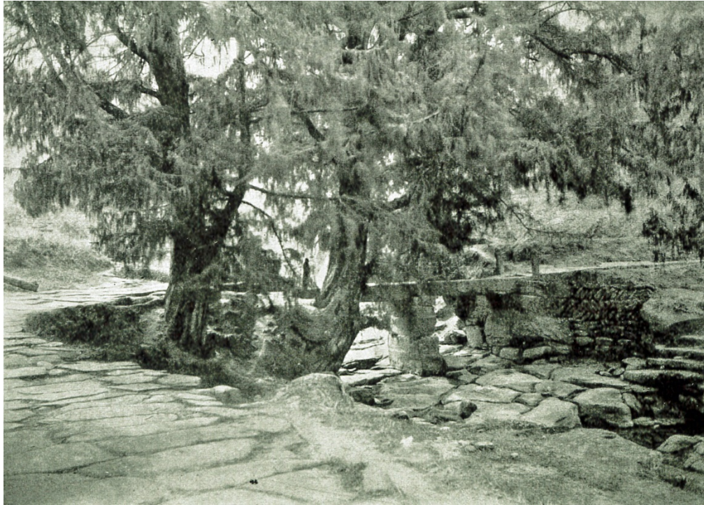
Figure 10 : Ancient bridge photographed north of Pu'an Zhen in Sichuan in 1897. Bridges like this can still be found in this area today. (From [R.25])
