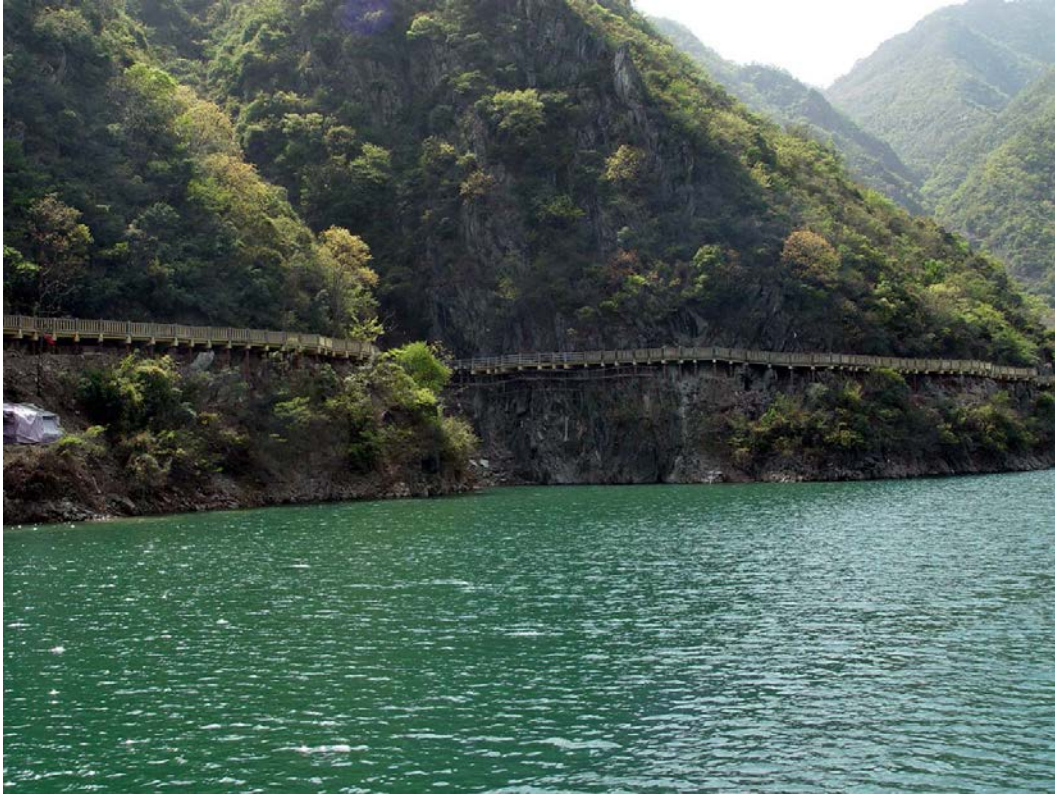
Reconstruction of the Plank Road at the Stone Gate Dam
