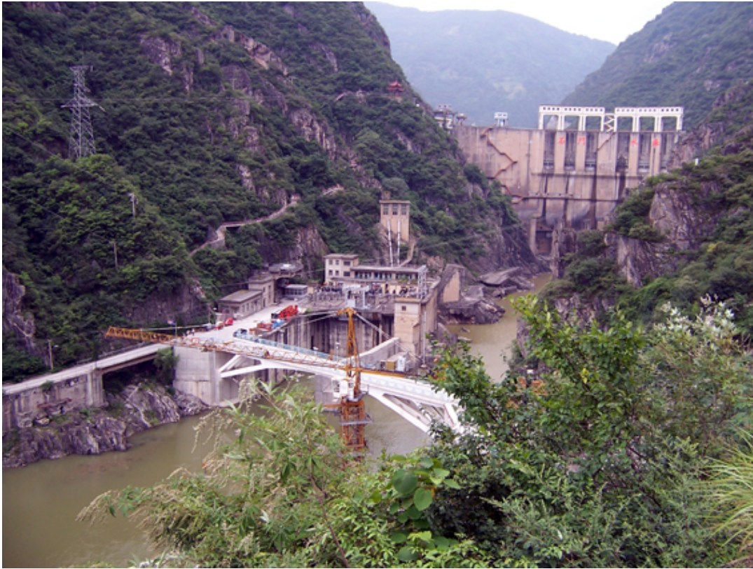
Stone Gate Dam Wall. Work continues.
